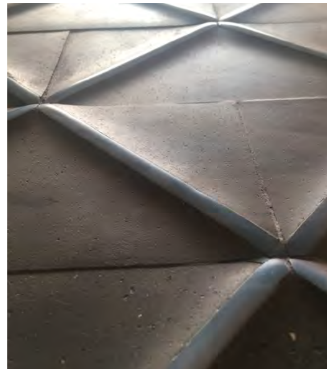
SURFACE DETAILS: THE GLASS WIDTH IS 6 MM - 2/8 THE RELIEF OF THE SAME IS 2/8 - 5 MM APPROXIMATELY.
